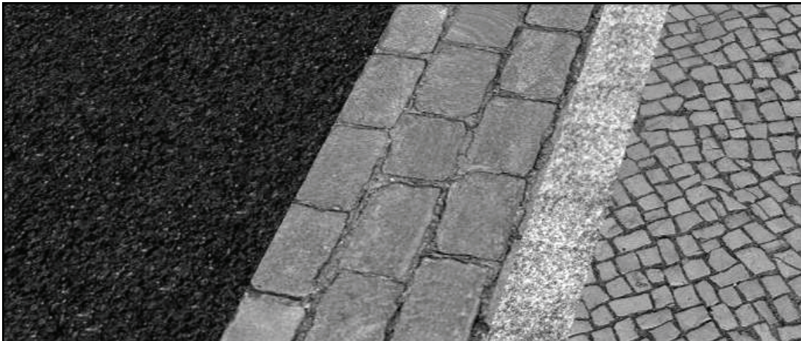
Figure 16: Examples of kerbs along the border lines of streets and sidewalks.
